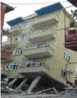
'Soft story' failure even in modern construction
