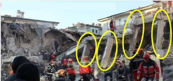
'Soft story' failure even in modern construction
