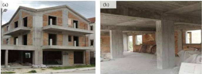
Example construction with shear walls and strong beams
